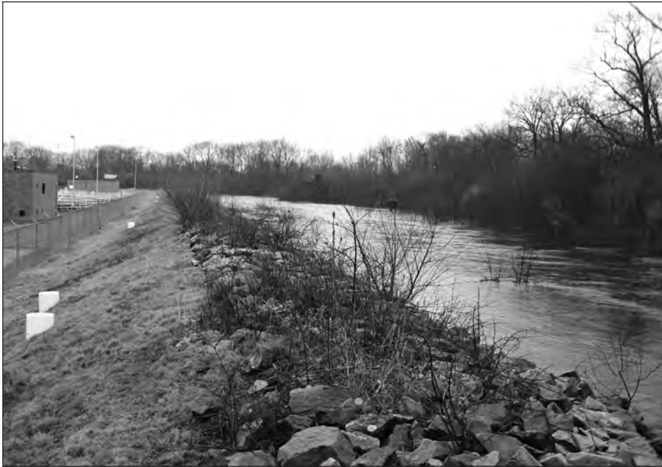
Figure 3 - Western Side of Levee at Warwick Wastewater Treatment Facility, March 15, 2010.
