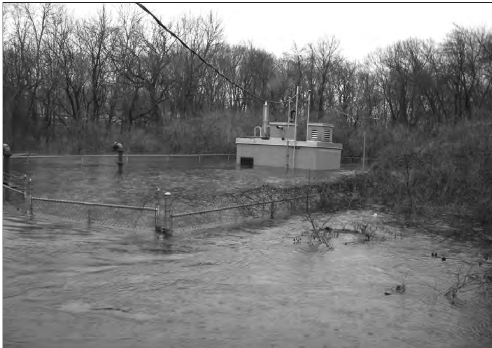
Figure 4 - Knight Street Pumping Station, located in a Pawtuxet River floodway, during The Little Flood. The station was designed like a submarine to operate in flood conditions. Note the smoke visible from the generator smokestack. This station pumped a lot of river water to the treatment plant before it was shut down in The Big Flood. Photo by Patrick Doyle
