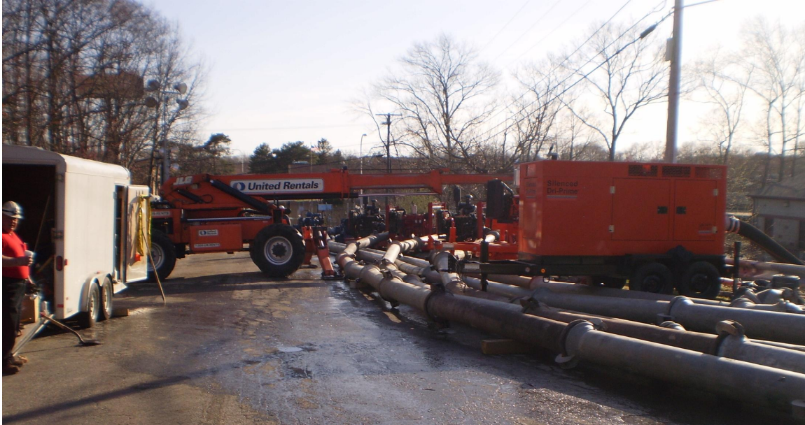
Figure 6: Portable Pumps Dewatering the WWTF Site. Photo by Janine Burke.
