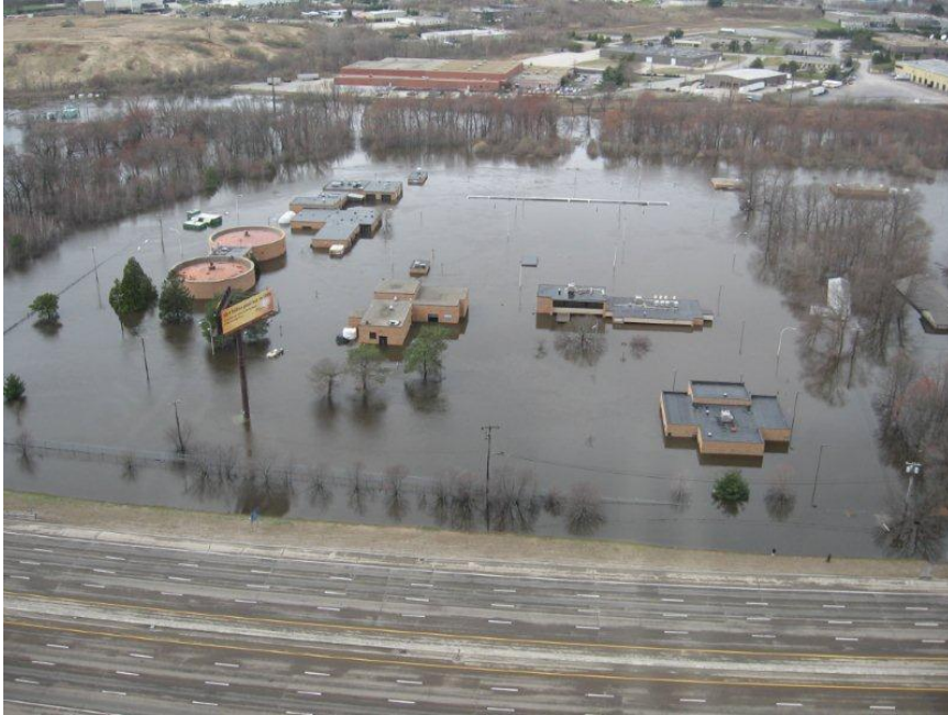
Figure 5: Flooding at the WWTF on April 1, 2010. Photo by Janine Burke.
