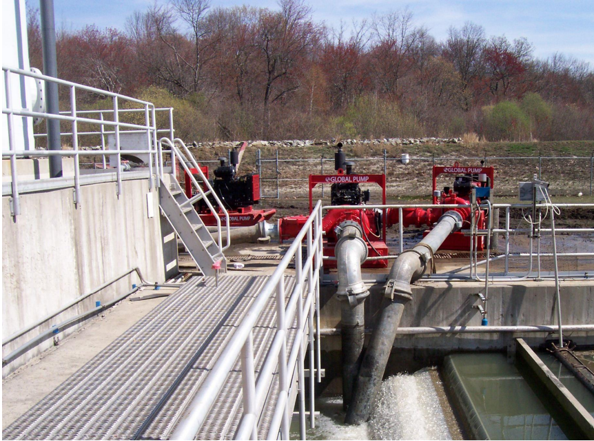
Figure 7: Portable Pumps Pumping Effluent. Photo by Erik Meserve.
