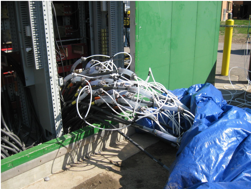
Figure 12: Nitrogen Gas Drying Manifold. Photo by Ron Demers.
