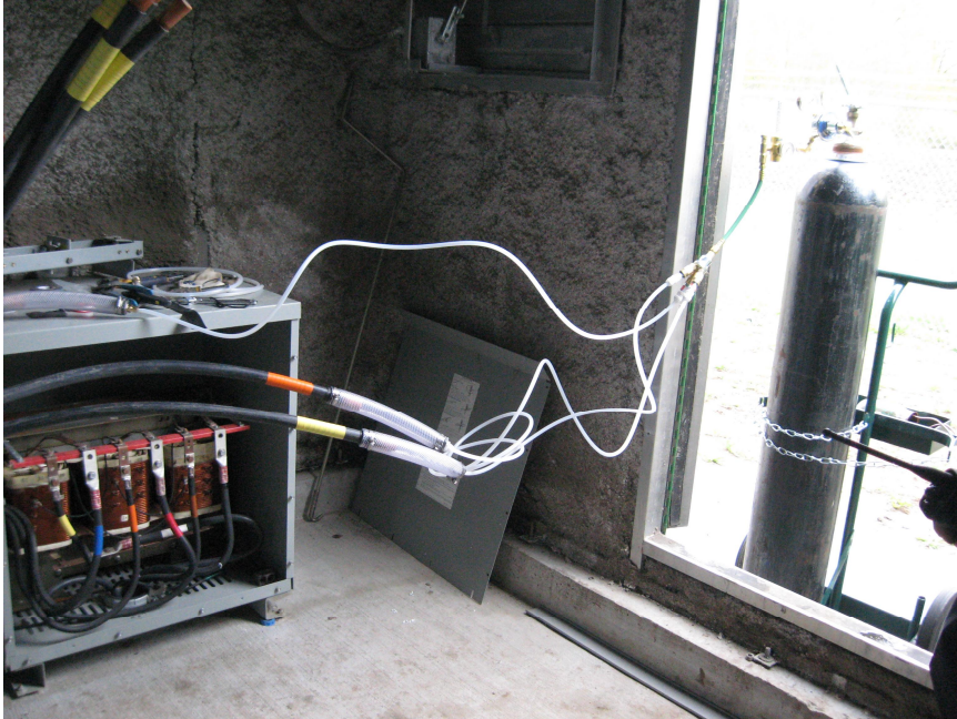
Figure 11: Nitrogen Gas Drying Test. Photo by Ron Demers.
