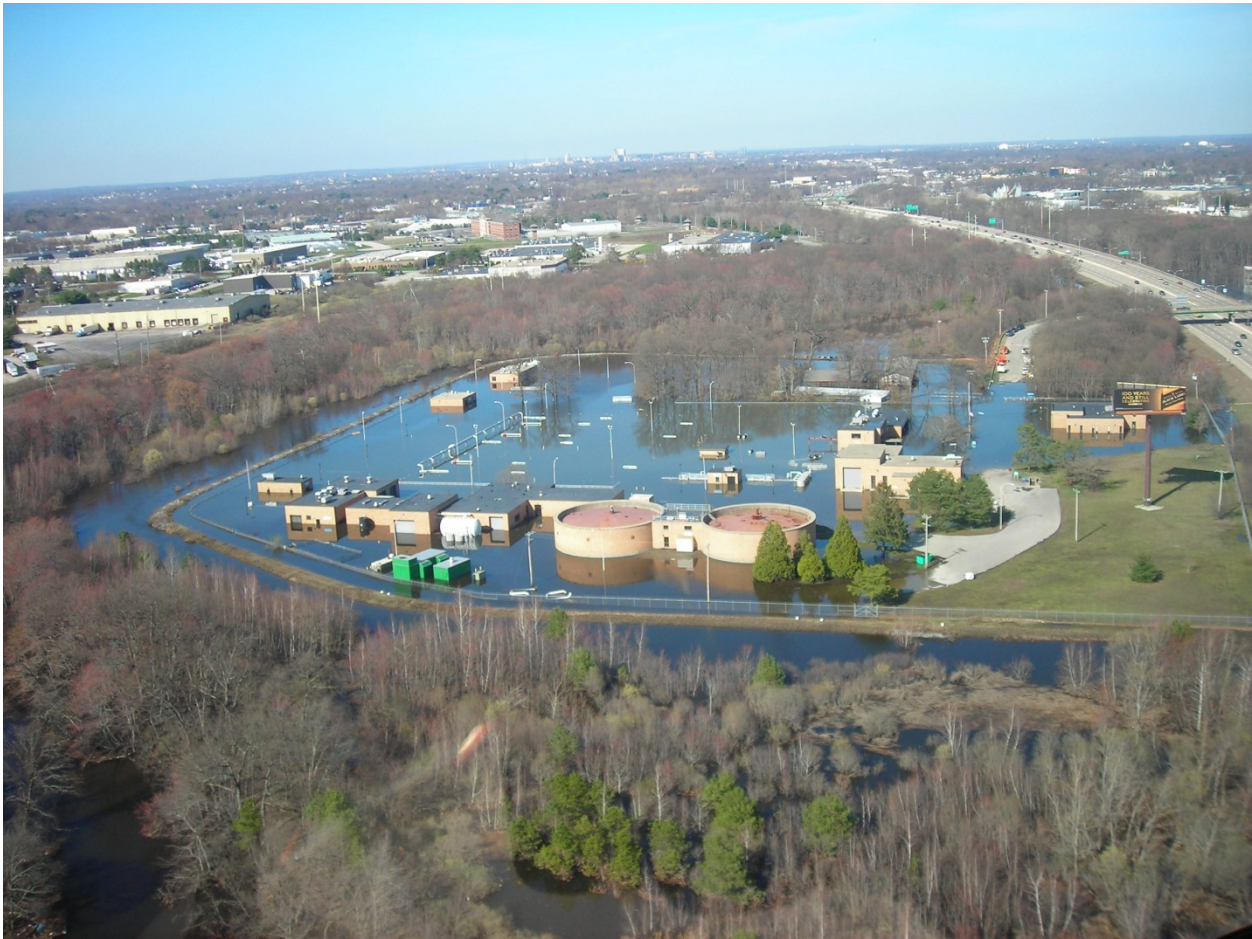
Figure II-3: Aerial Photo of Warwick WWTF, April, 2010
