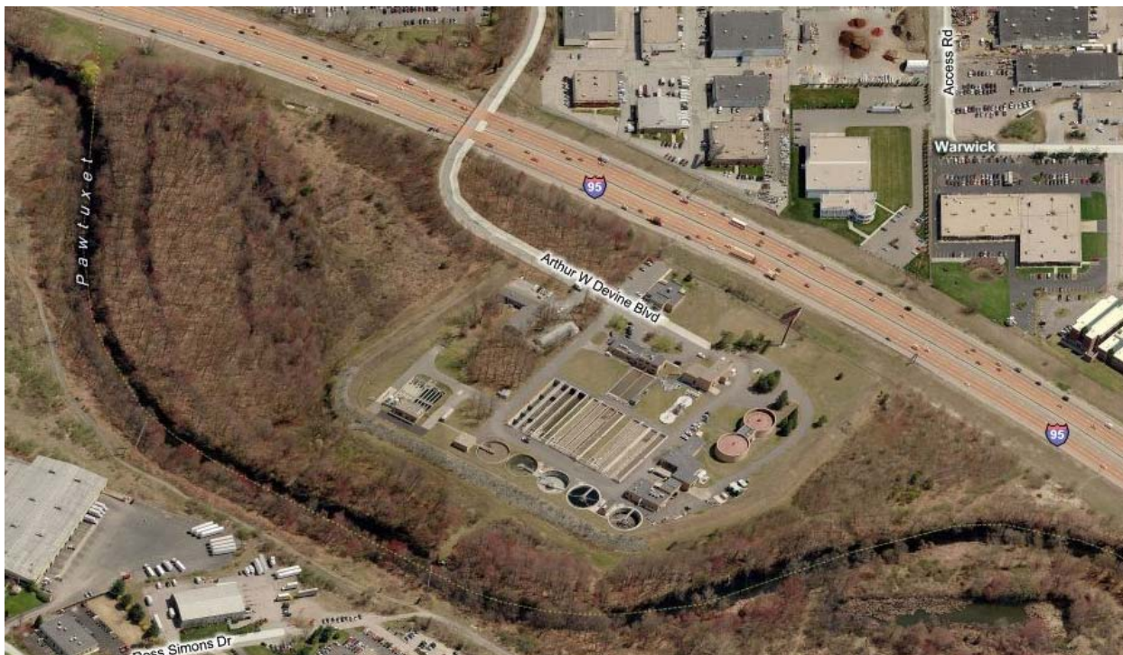
Figure II-1: Aerial of Warwick WWTF
