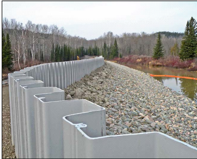
Figure V-2: Example Vinyl Sheet Pile Wall
